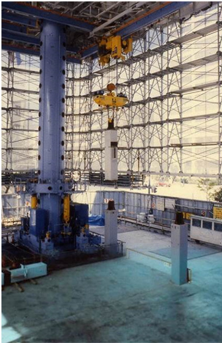
Fig. 4. The concept of robot-oriented design applied in an automated construction site (SMART) of the company Shimizu.
